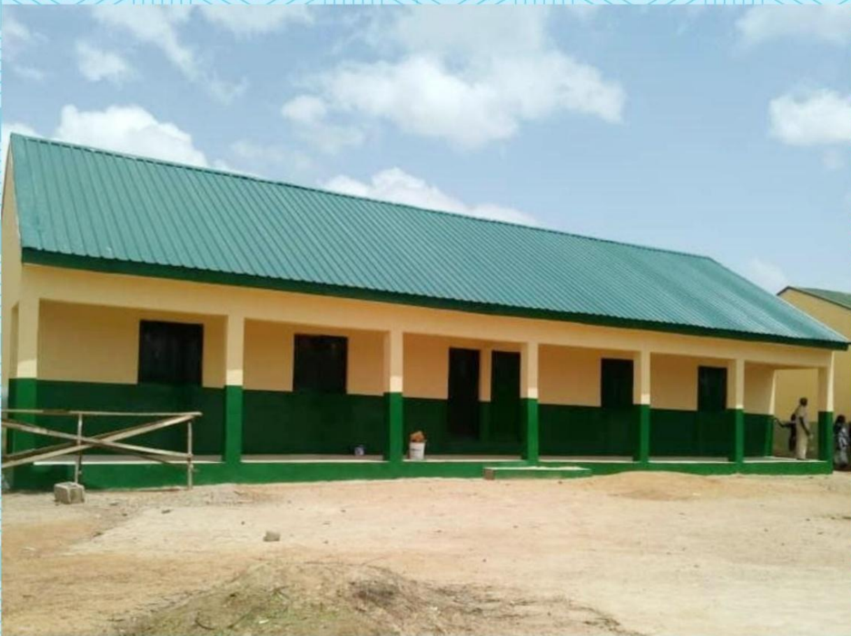
Works in progress
